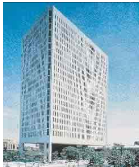
Fig. 5 Window Wall Panels Serve as Elements Of Vierendeel Truss on One Hundred Washington Square Office Building, Minneapolis, Minnesota [9]
