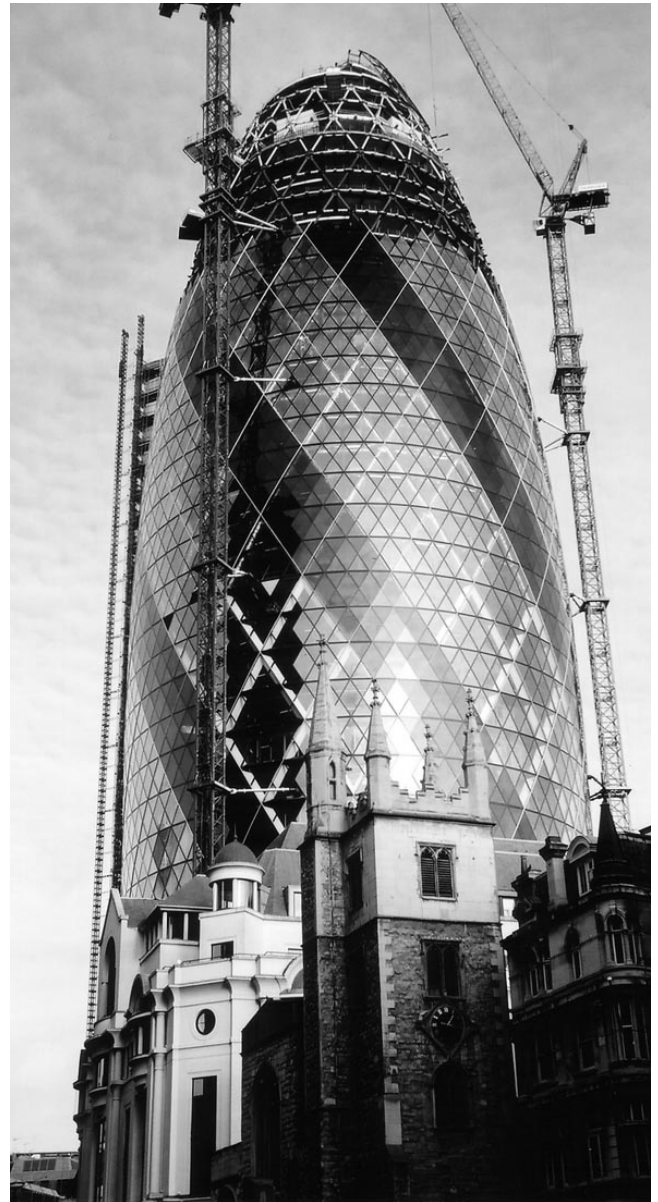
Figure 9: 30 St. Mary Axe during construction (Courtesy of John E. Fernandez).
