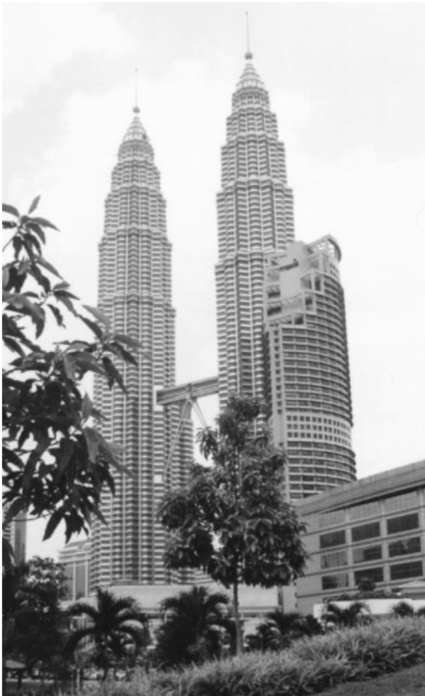
Figure 14: Petronas Tower (Courtesy of Abbas Aminmansour).
