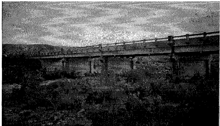
Figure 3 Alamosa Canyon Bridge.
