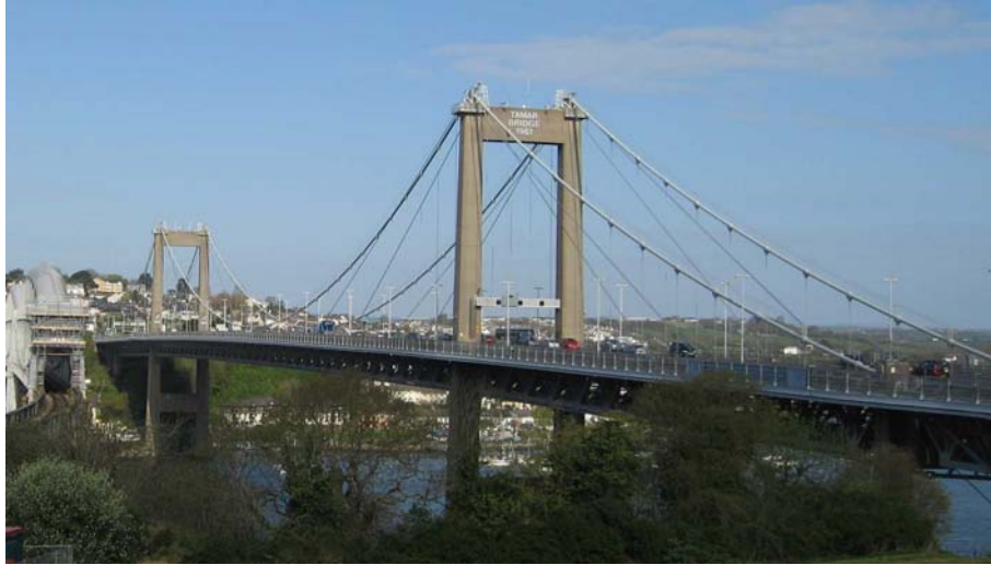
Figure 1: Tamar suspension bridge
