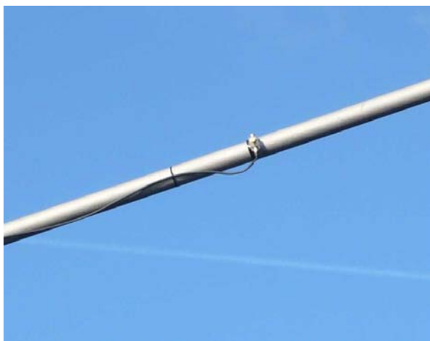
Figure 14: Biaxial accelerometer on stay cable.
