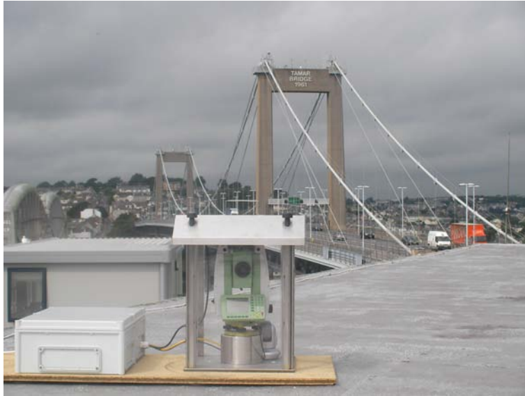
Figure 31: TPS for Tamar Bridge Monitoring
