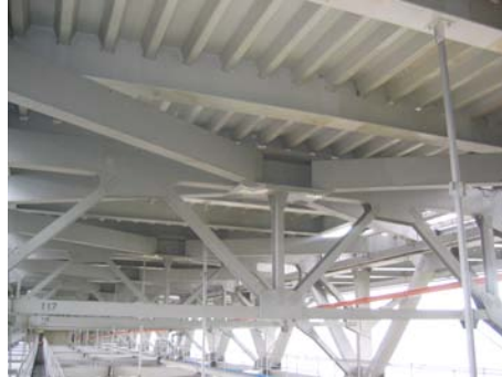
Figure 6: Orthotropic main deck
