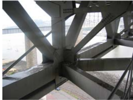
Figure 3: Deck truss and additional longitudinal girder
