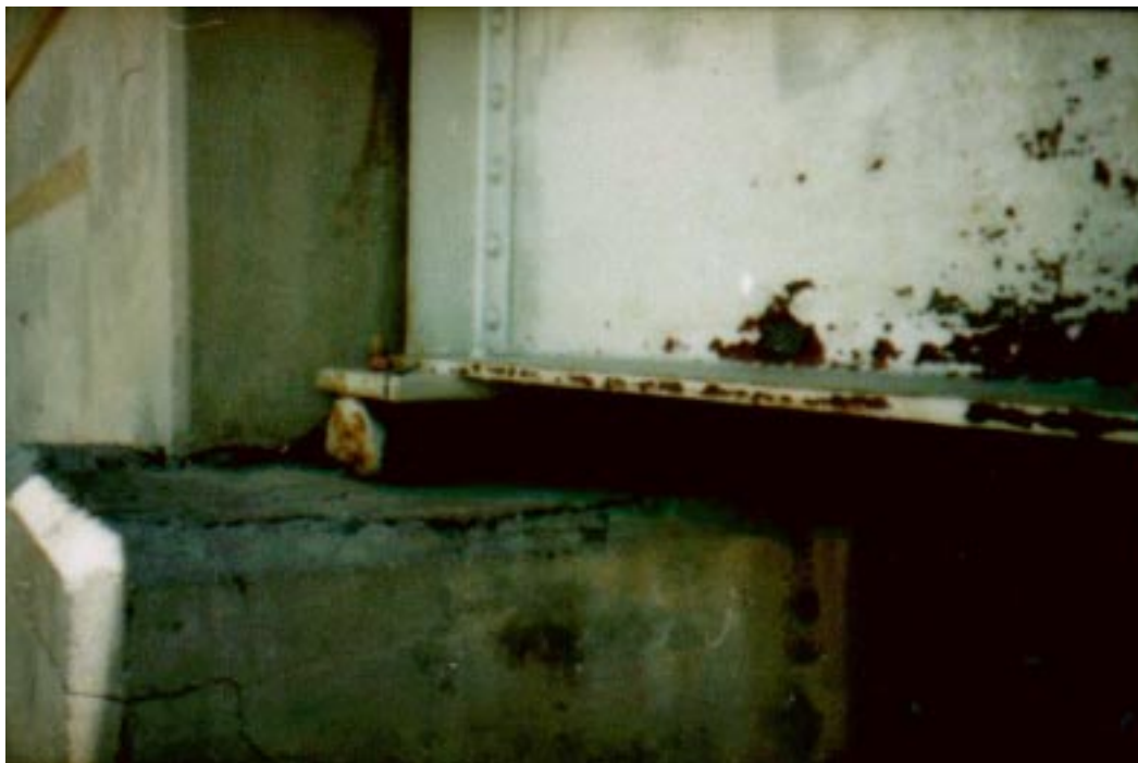
Figure 11. Photo of a half-roller connection at the northern abutment.
