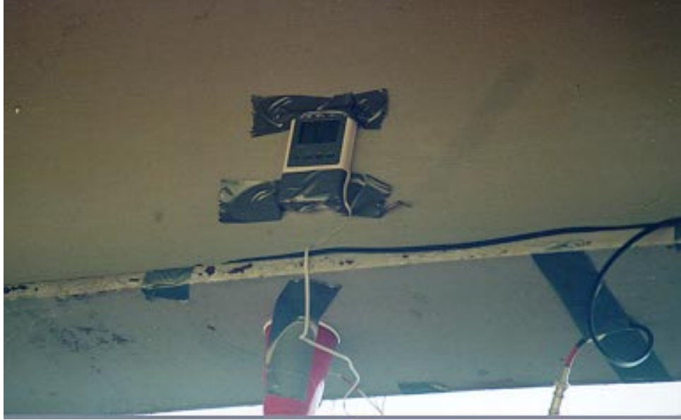
Figure 34. Indoor-outdoor thermometer taped to the exterior girders.
