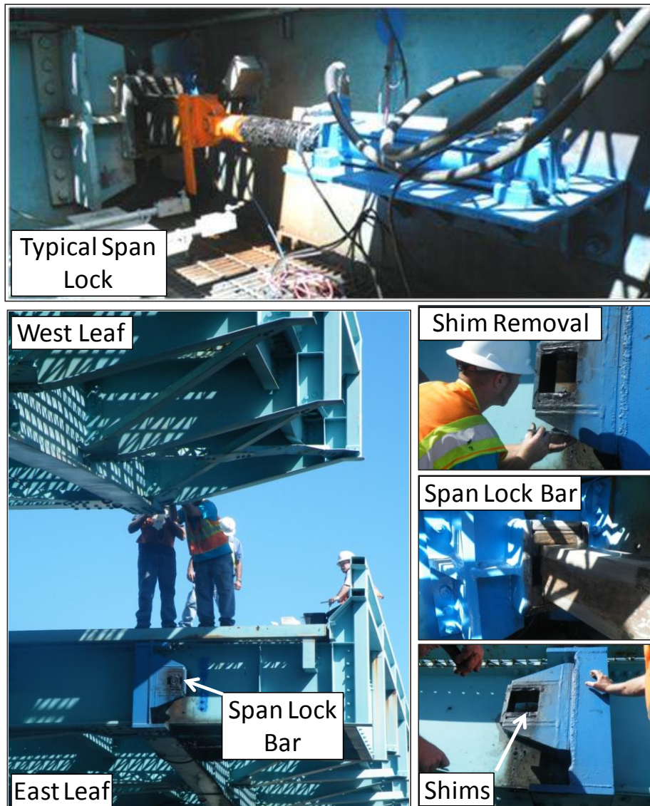
Figure 38: Span lock (SL) and the shim removal operation
