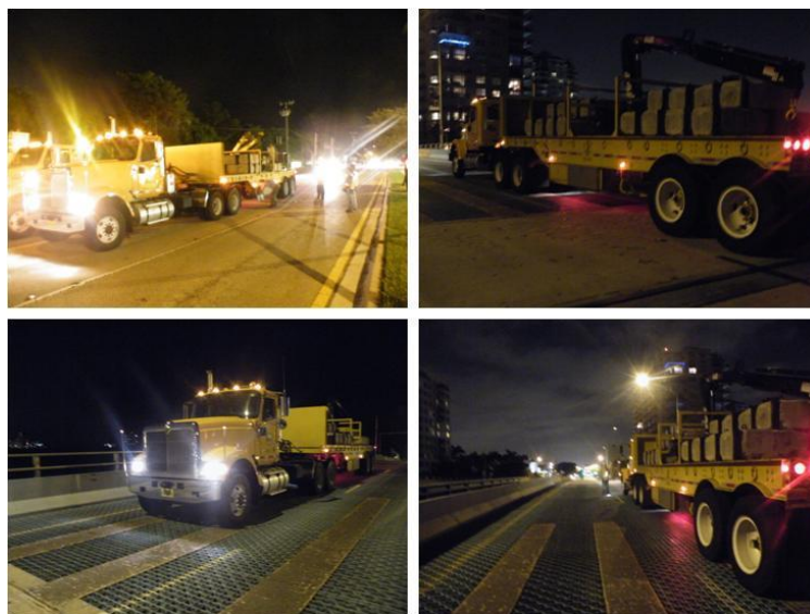
Figure 18: Truck load test on Sunrise Boulevard Bridge
