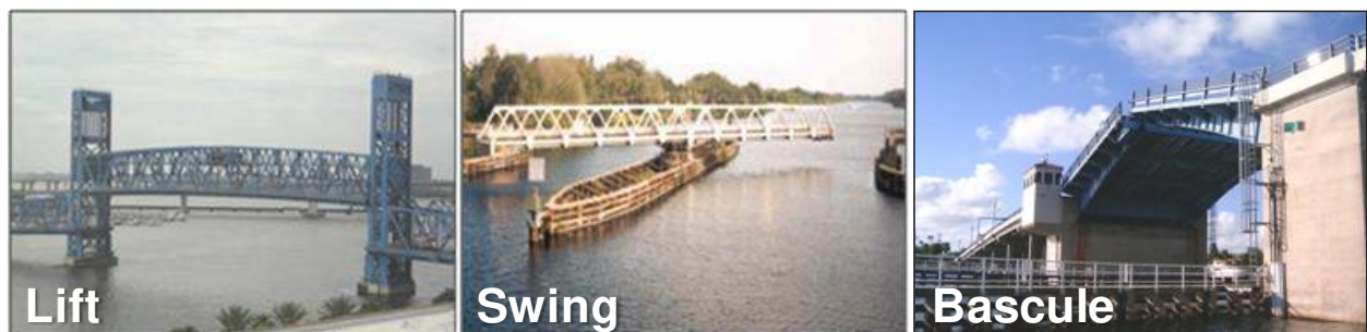
Figure 3: Main types of movable bridges
