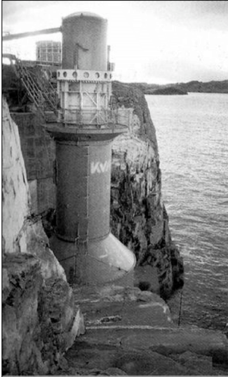
Figure A.2: The shoreline OWC device in Toftehallen, Norway, built into a cliff.
