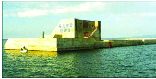
Figure A.3: Breakwater of the port of Sakata, Japan, with an integrated OWC device.
