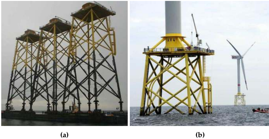
Fig. 1.2: (a) OWEC jacket being transported to Alpha Ventus, Germany. (b) Senvion 5 MW turbines installed at Alpha Ventus. Courtesy of offshorewind.biz and power-technology.com.
