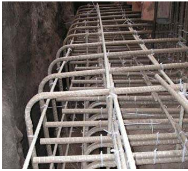
Fig. 1. Use of GFRP bars in retaining wall in coastal bluff: site (a), and reinforcement cage (b). Credit: Hughes Brothers.
