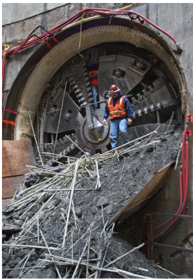
Fig. 2. Use of GFRP bars in soft clay: installation of wall reinforcement (a), and TBM breakthrough (b). Credit: Hughes Brothers (a), and Jacobs Engineering Group (b).
