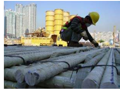
Fig. 3. GFRP #10 bars: closeup (a), and soft clay cage under construction (b). Credit: Hughes Brothers (b).
