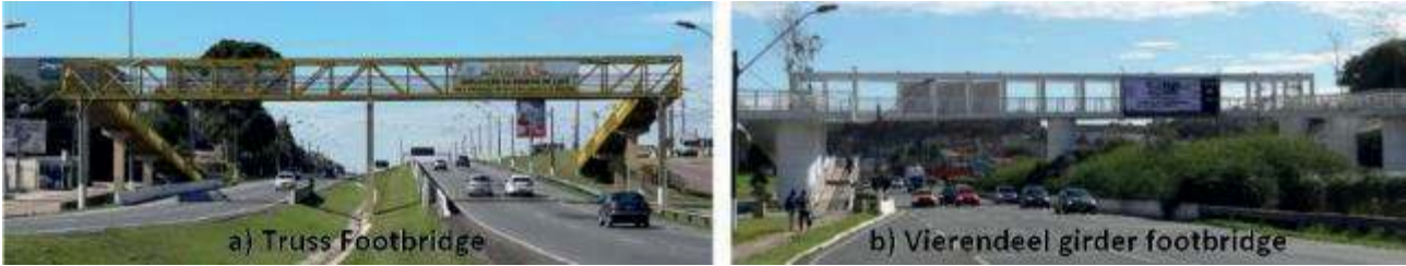
Figure 14. Typologies of existing footbridge on the highway under study.
