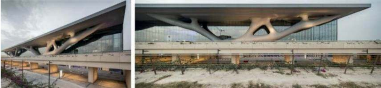
Figure 7. Qatar National Convention Center.
