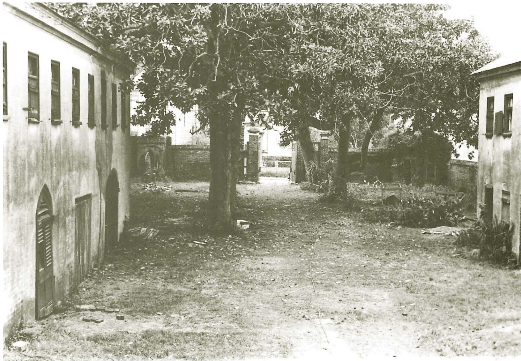
Figure 13.4: View of the back yard of the Aiken-Rhett site. The structure to the left is stables and groomsmen quarters; the building on the right served as a kitchen, with slave quarters above. Excavations focused on the rear portion of the yard behind these outbuildings.
