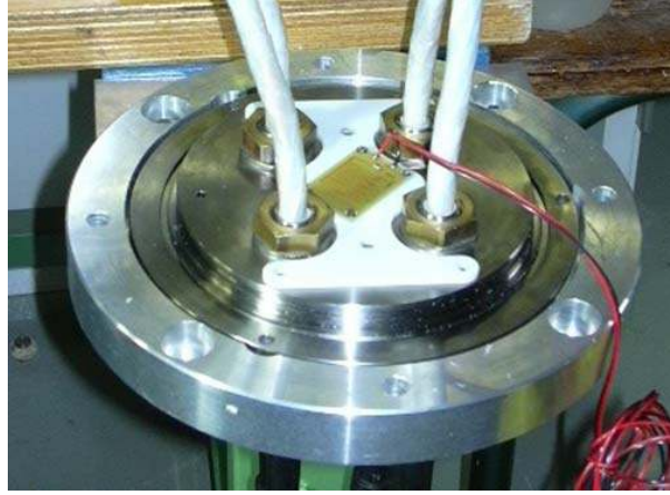
Fig.7b. Leak sensor installation on the optical module connector flange.
