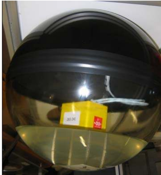
Fig. 7c. TinyTag installation in an optical module sphere.
