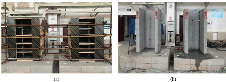
FIGURE 10: Fabrication and formation of walls. (a) Formwork support. (b) Specimen shaping.
