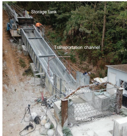
Figure 2. Flume facility (with Barrier 2 installed)
