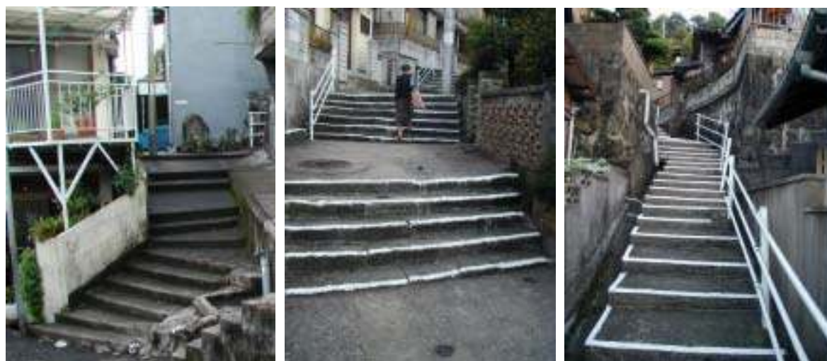
(a) highly irregular stairs
