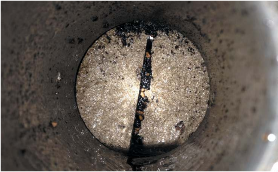
Fig. 13. Fracture opening (1 mm) partially plugged
