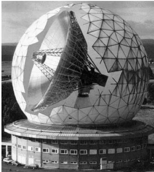
Figure 4: FGAN Tracking and Imaging Radar (TIRA). Source: [1]
