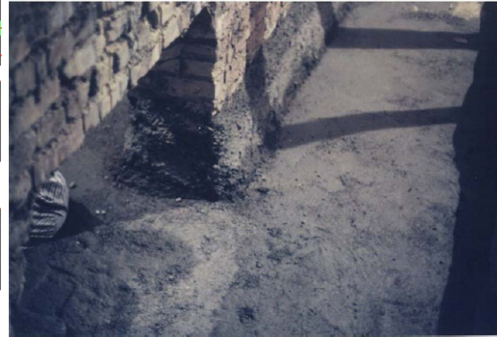
Figure 5: Performing of a Khorjini Foundation
