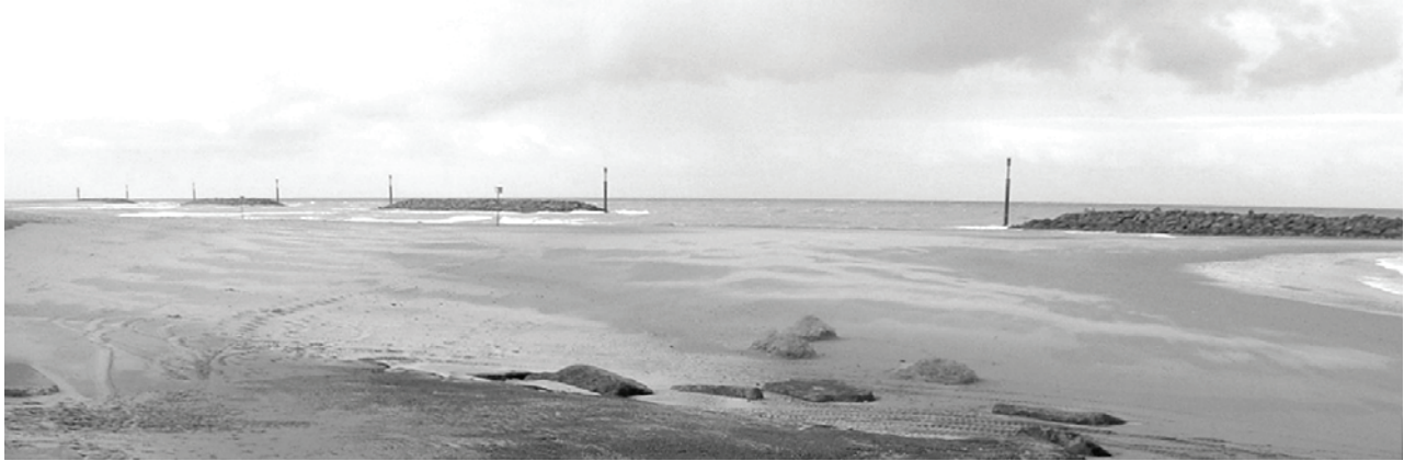
Figure 1. The northernmost four shore-parallel breakwaters at Sea Palling in East Anglia, UK.
