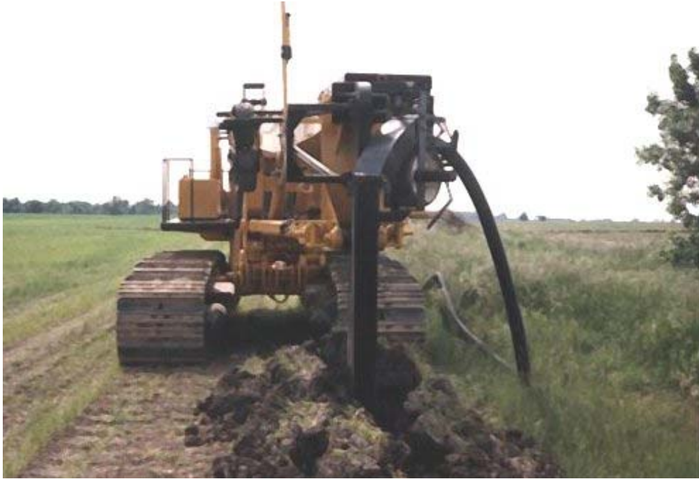
Figure 4. Laser controlled plow installation of plastic drain lateral.
