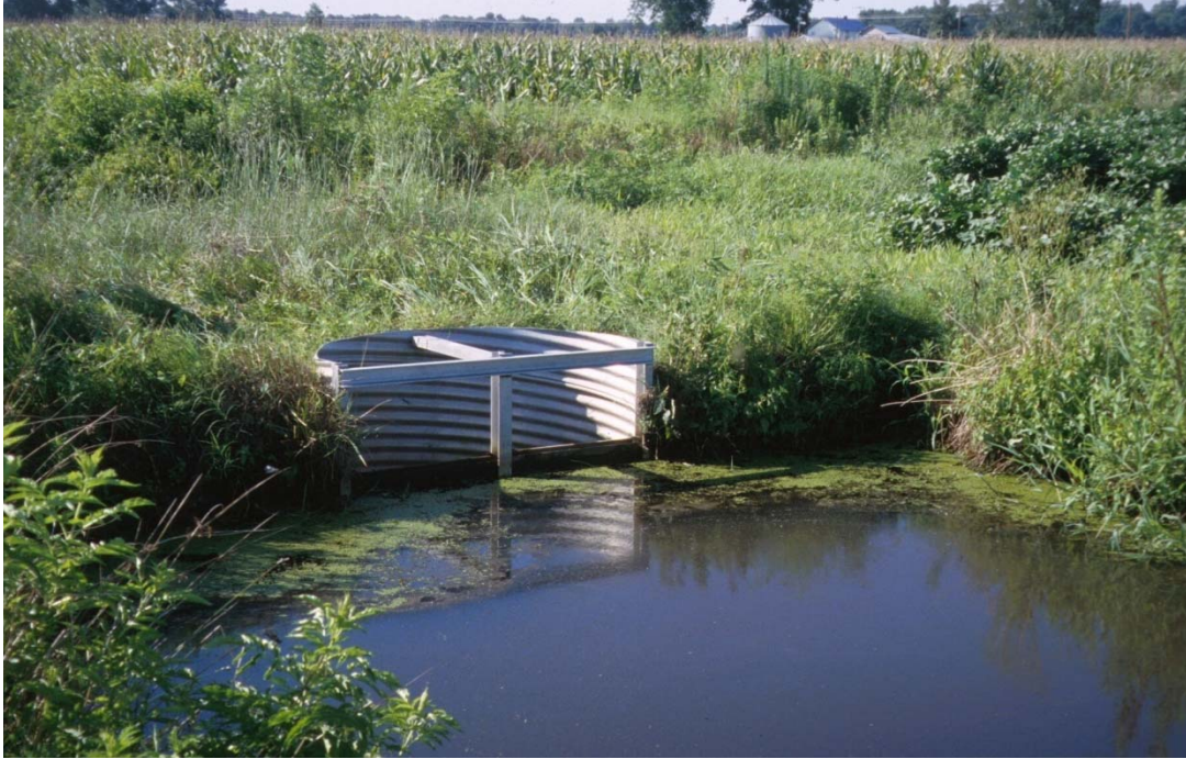
Figure 6. Drainage control structure in humid region.
