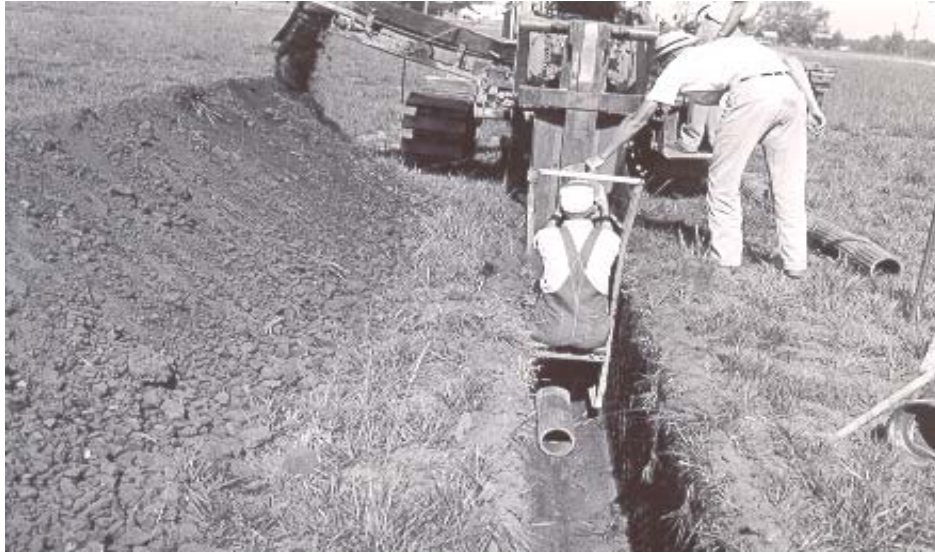
Figure 2. Hand installation of drain tile.
