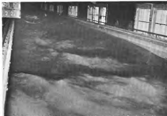
FIGURE 25.—Upstream view of the water surface in the area of antidune activity during run 18.
