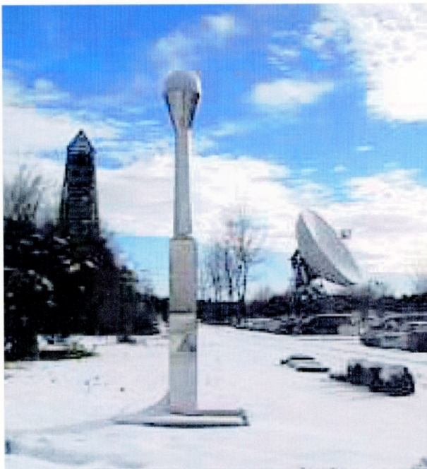
FIG. 9. GPS network sites in Japan are housed in 5-m tall stainless steel towers, as shown. The sites are maintained by private companies under contract; communications are provided by telephone.
