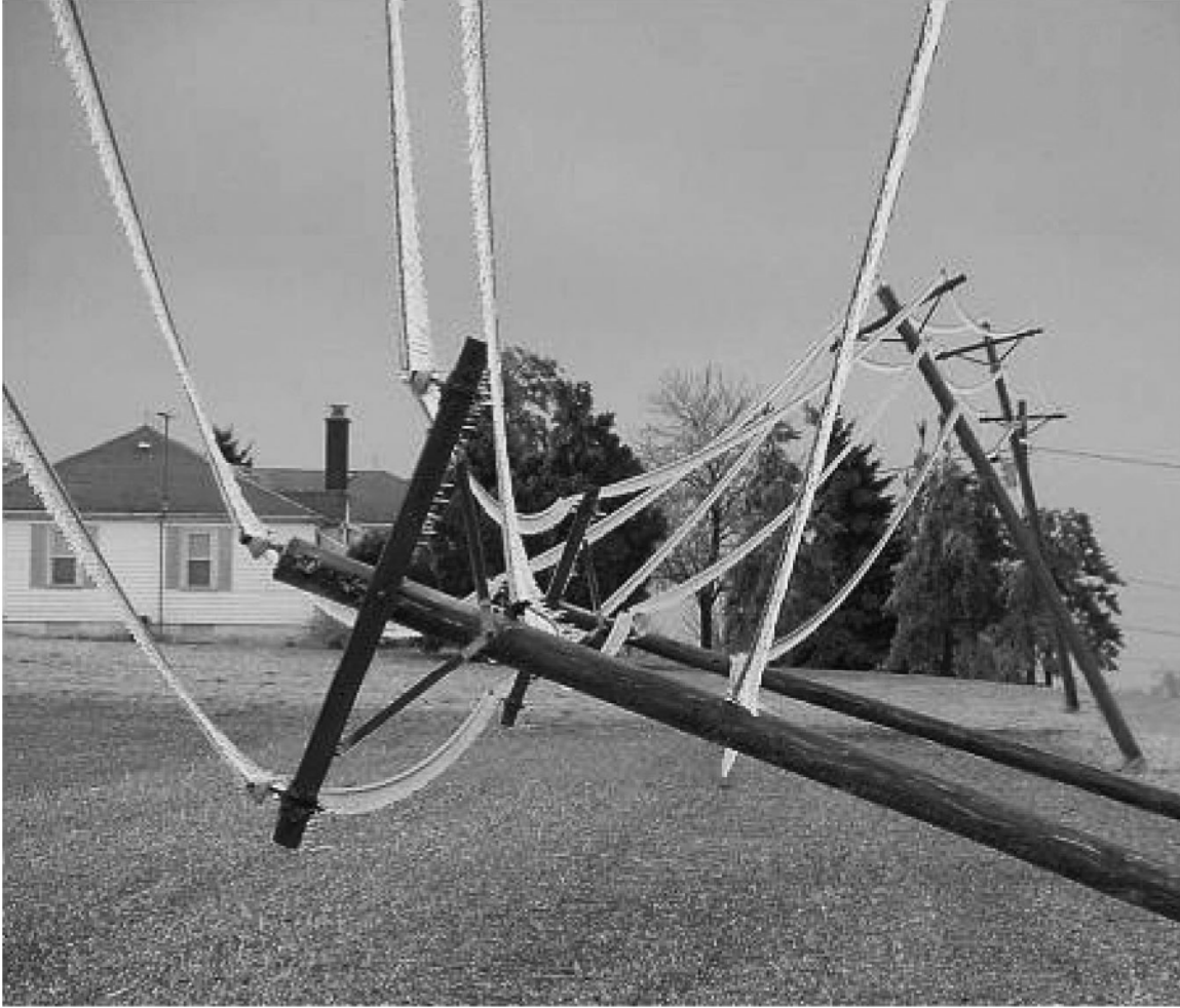
Figure 1. Image of fallen wood poles due to ice deposited on metal cables.
