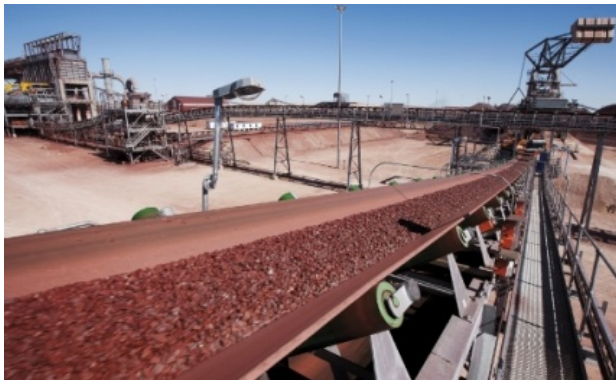
Figure 1.1: Handling of iron ore using a belt conveyor at Kolomela mine [2].
