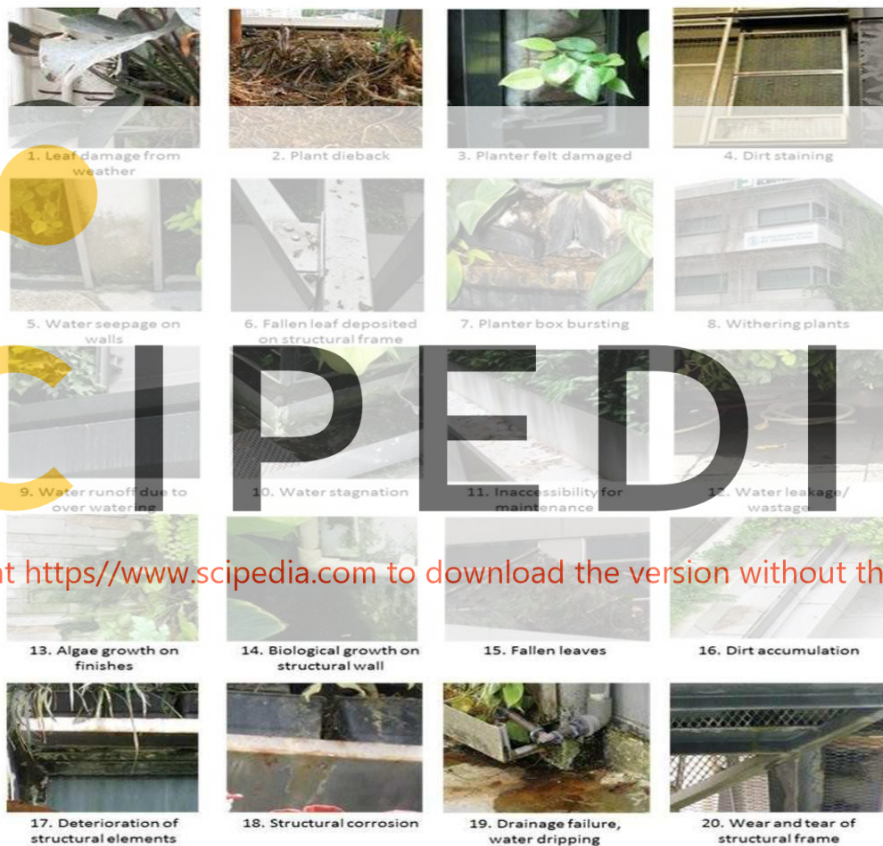
Figure 1. Some Defects of Vertical Greenery Systems. (Source: Chew and Conejos, 2016).
