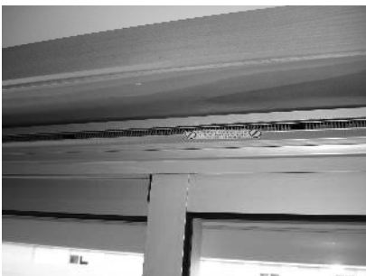
Figure 7. Ventilation grids on window frames.
