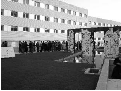
Figure 1. General exterior view of the building blocks.
