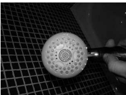
Figure 5. Low flow showers.
