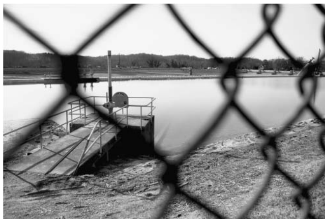
Figure 5. A sewage treatment plant outside Washington, DC, behind a chain-link fence, emblematic of the societal stigma associated with what is actually a resource: excreted phosphorus. Photograph: Craig Brown.
