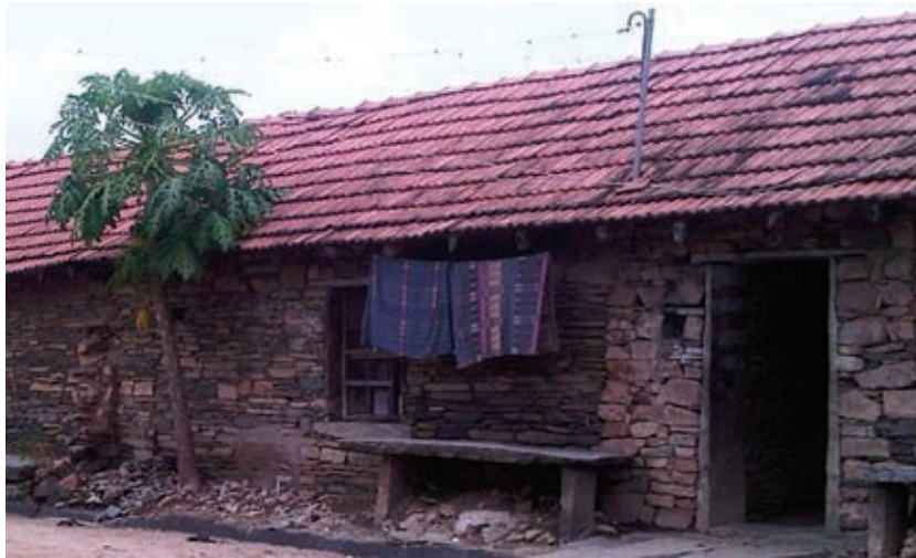
Figure 9: Traditional single-storied dwelling (stone walls, clay-tile roofs).
