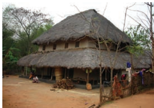
Figure 3: Traditional two-storied tribal shelter (earthen walls, thatch roof).
