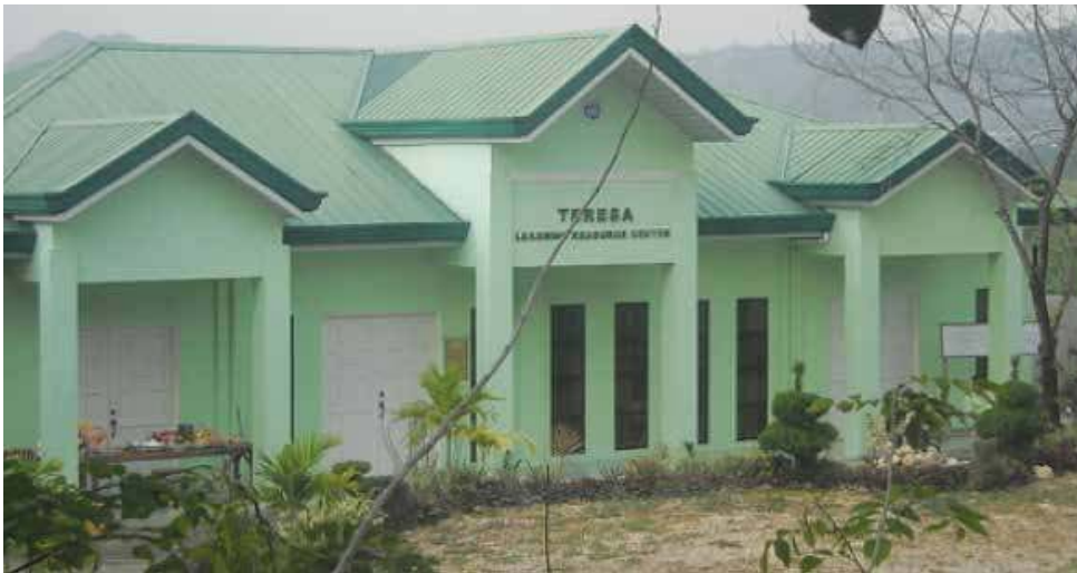
The Integrated Solid Waste Management Facility in Teresa, Philippines operates a Learning Resource Center where waste management training is offered to local government units and interested parties for a fee. Photo credit: Teresa Municipal Environment and Natural Resources Office
