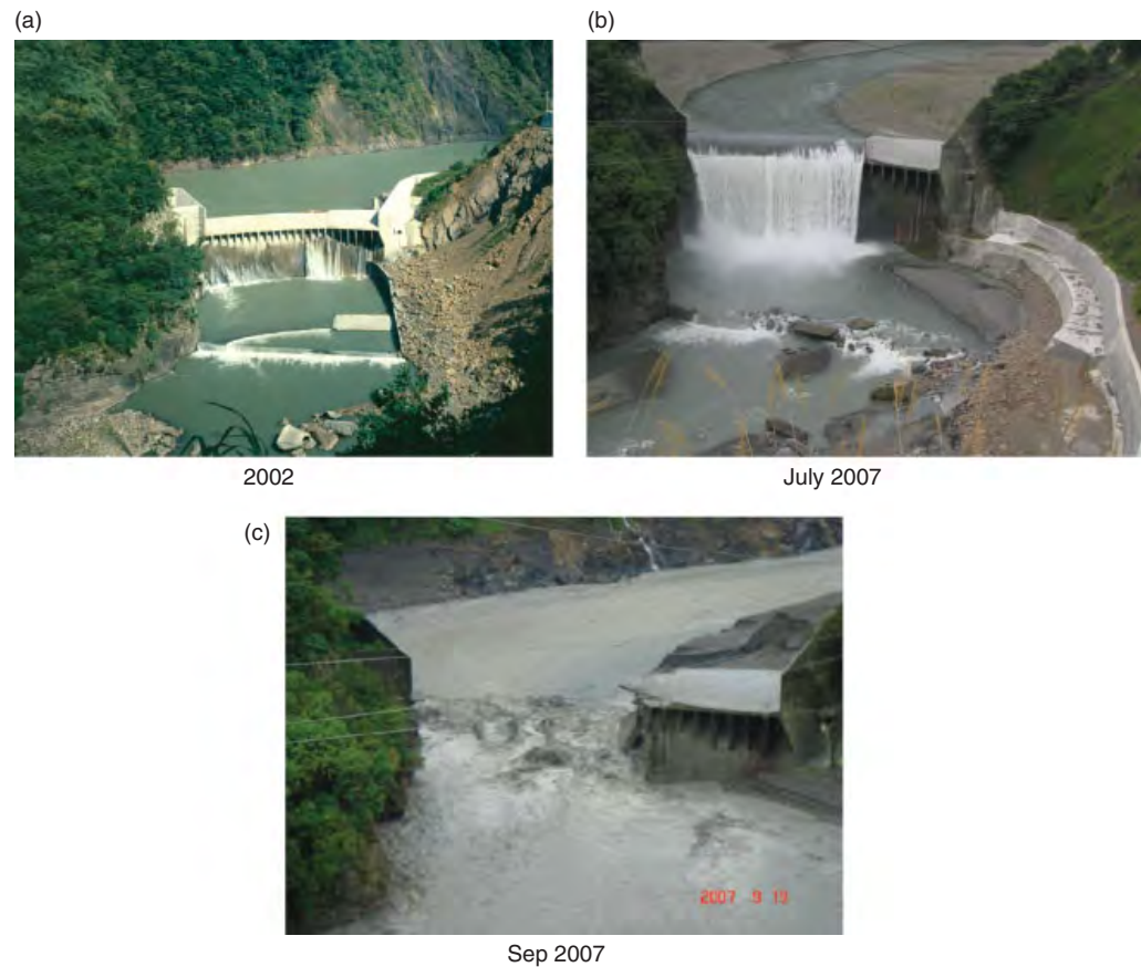
Figure 15. Sequential photographs looking at Barlin Dam, showing the dam (a) prior to filling with sediment (October 2002), (b) after filling with sediment (September 2005), and (c) after failure (September 2007). (Photographs courtesy of Taiwan Water Resources Agency, reprinted by permission.)
