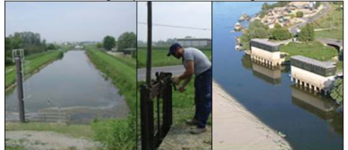
Fig. 3. Water distribution management pilot: open earth canal (left), manual operation (center) and water intake (right)
