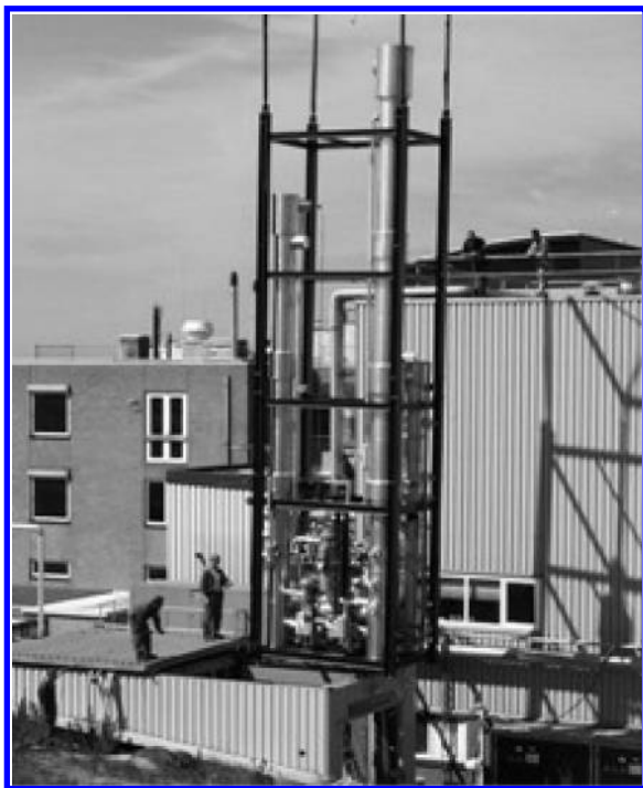
Figure 16. Mounting of the OLGA pilot installation at ECN.
