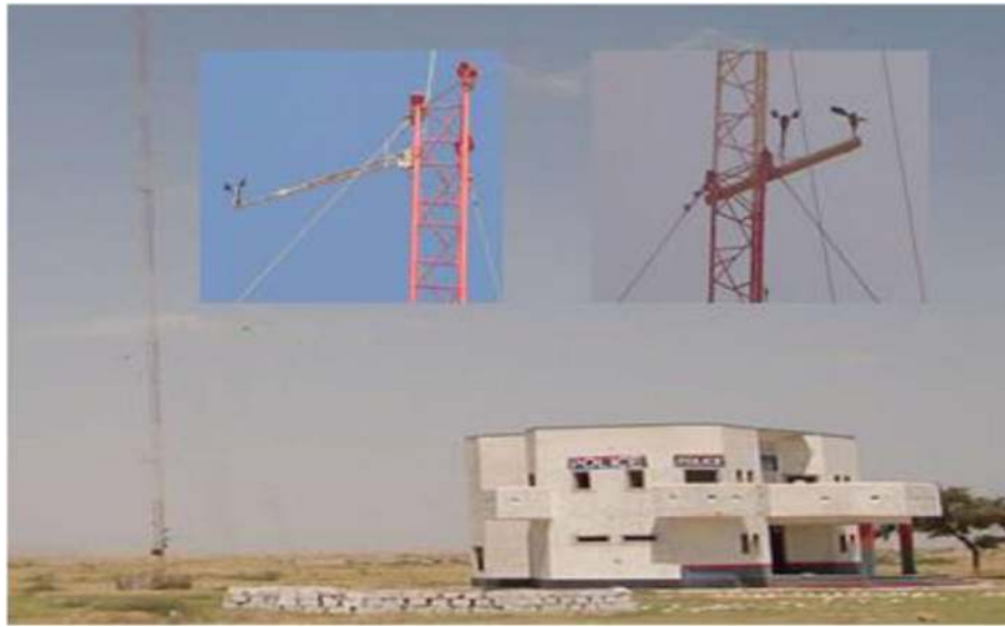
Fig. 4 Nooriabad Met Mast at Super Highway (mounted wind vane)
