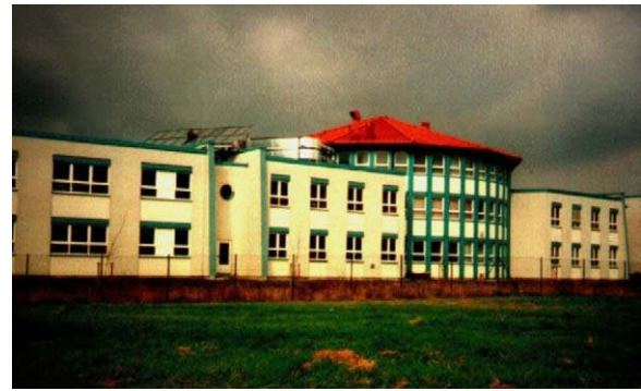
Fig. 17. Solar desiccant cooling system installed in Riesa, Germany [111].
