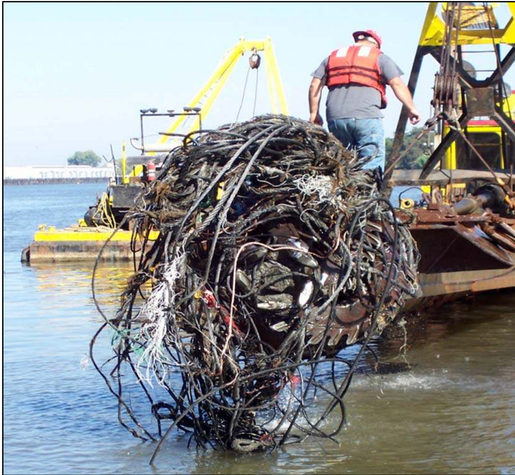
Figure 10. Debris fouling of cutterhead by cables.
