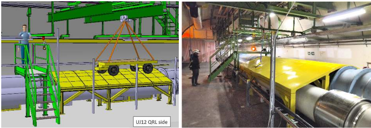
FIG. 24. The schematics of the transport setup at UJ12 (left) and a current photo of the site (right). The yellow QRL protection will allow us to transport \text{FASER}\nu even when the LHC is cold.
