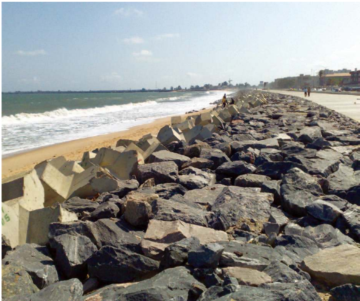
Figure 4.10: Bar Beach seawall, Victoria Island, Lagos, Nigeria
