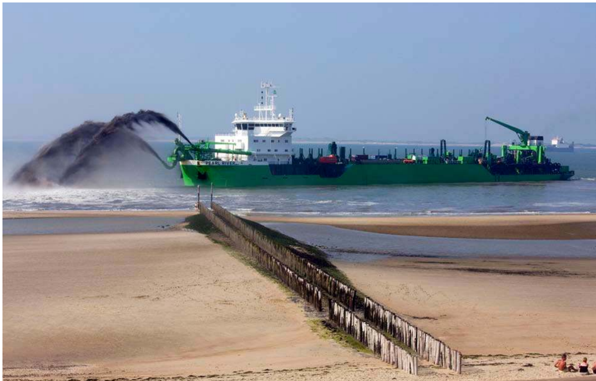
Figure 4.2: Rainbow method for transferring nourishment material ashore
