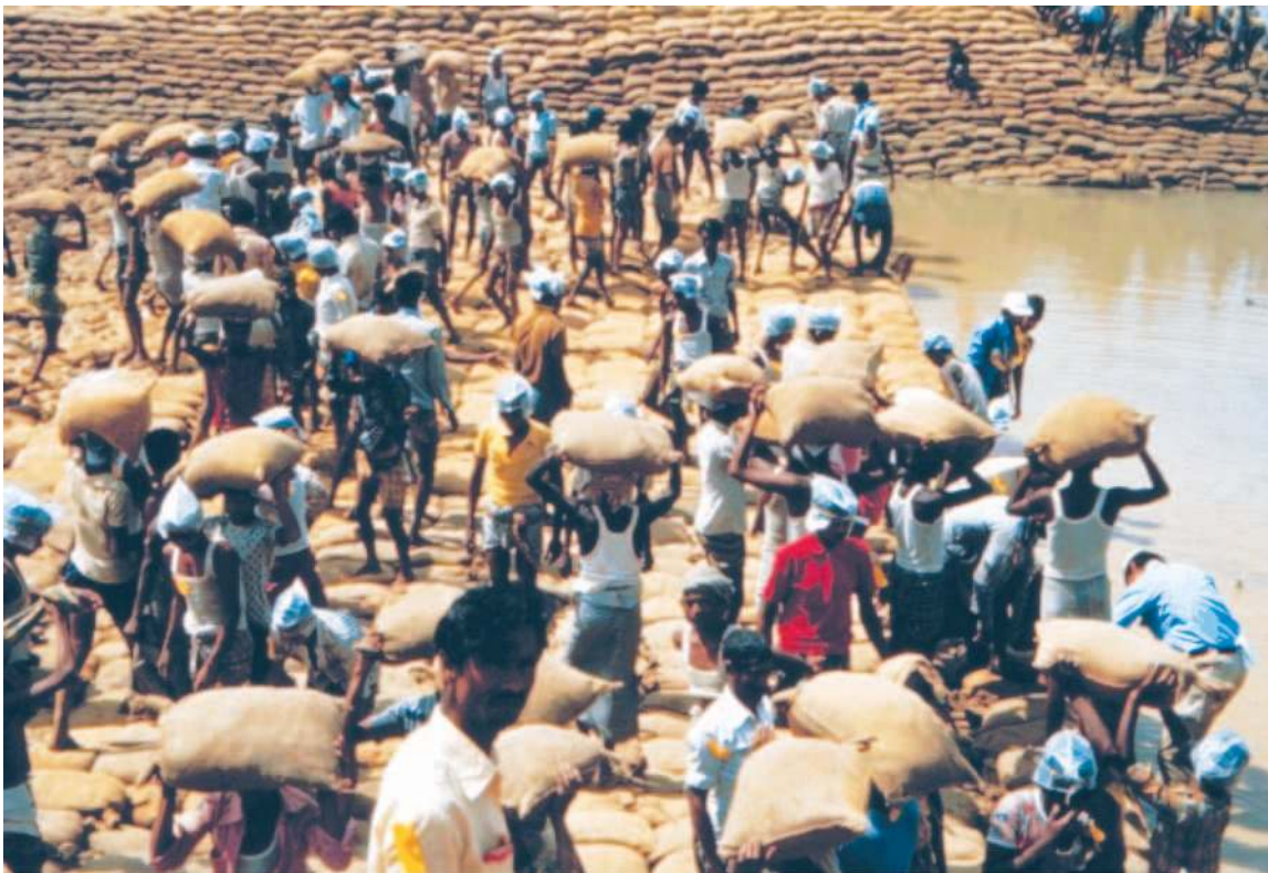
Figure 4.16: Closure dam under construction at Jamuna river, Bangladesh
