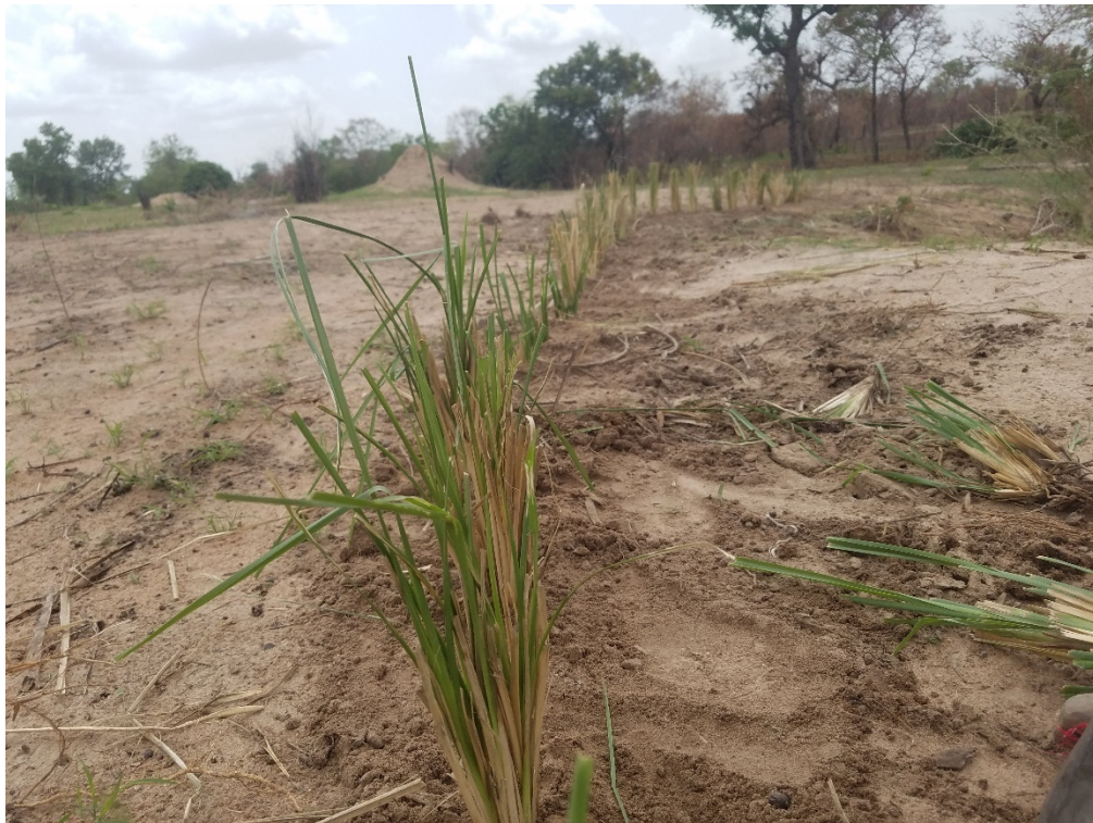
Figure 18. Vetiver grasses spaced out at 20cm spacing along the bank (photo by author).
