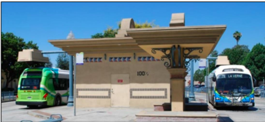
Figure 12. Charging station for the Proterra Bus [20]
