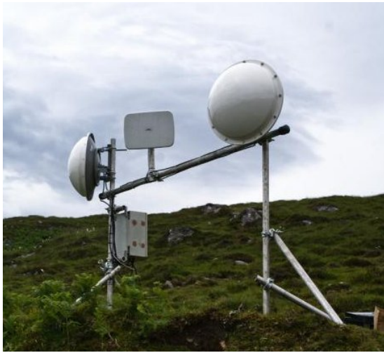
Figure 3: Mast at node K in Figure 1, illustrating our current approach to mast construction.
