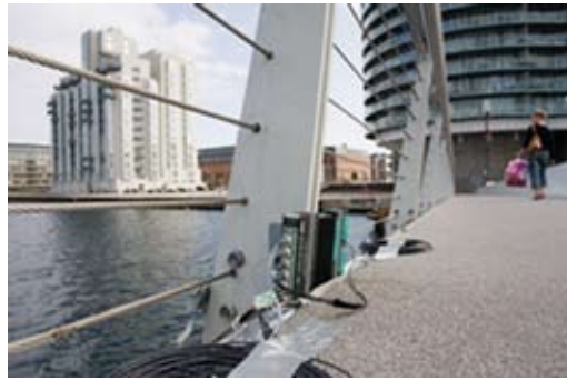
Figure 5: Bridge vibration monitoring. Photo courtesy of Bruel & Kjaer.
