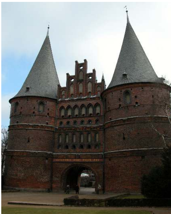
Figure 2. Western facade front of the Holstentor, Lübeck
