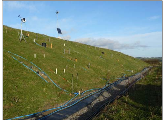
Figure 1. Full-scale test embankment.
