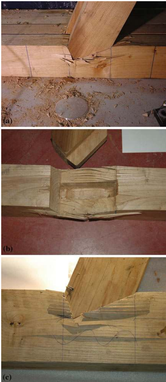
Fig. 4 Typical experimental failure patterns observed: a joint collapsed in compression, with uniform distribution of damage, b joint collapsed in compression, with out-of-plane bulging, and c combined failure in compression and shear parallel to the grain at the toe
