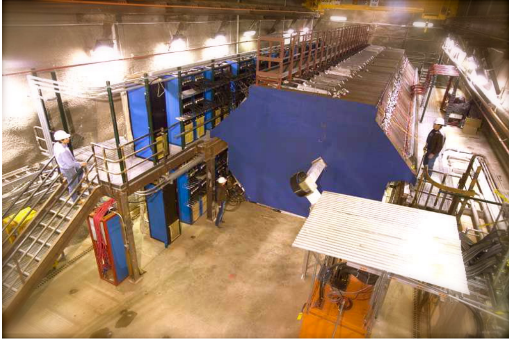
Figure 4.9: The MINOS Near Detector. The blue plain is plane zero of the ND with the rest of the detector behind it. The racks holding the electronics are seen on the ground and the walk way on the left of the detector. The white structure in-front of the detector is ArgoNeuT.
