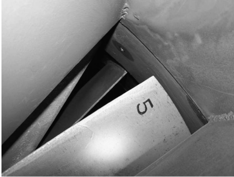
Figure 8.—Probe installation on the axial vane fan.
