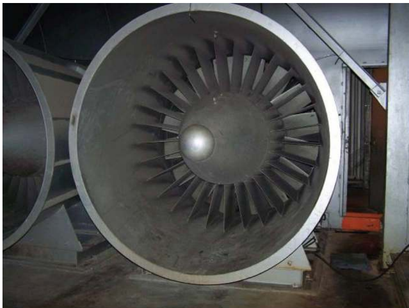
Figure 7.—Axial vane fan located at the 10 \times 10 SWT.
