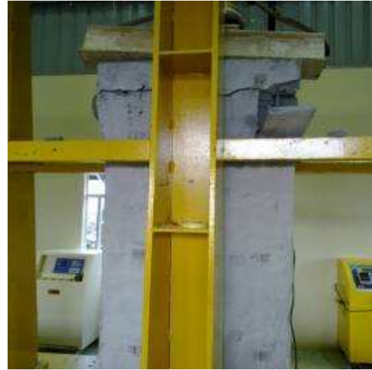
Fig. 23: Cracking at Top Part of Panel 2
