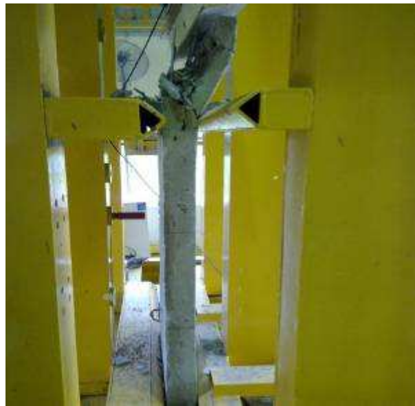
Fig. 24: Crushing at the Top Part of Panel 2
