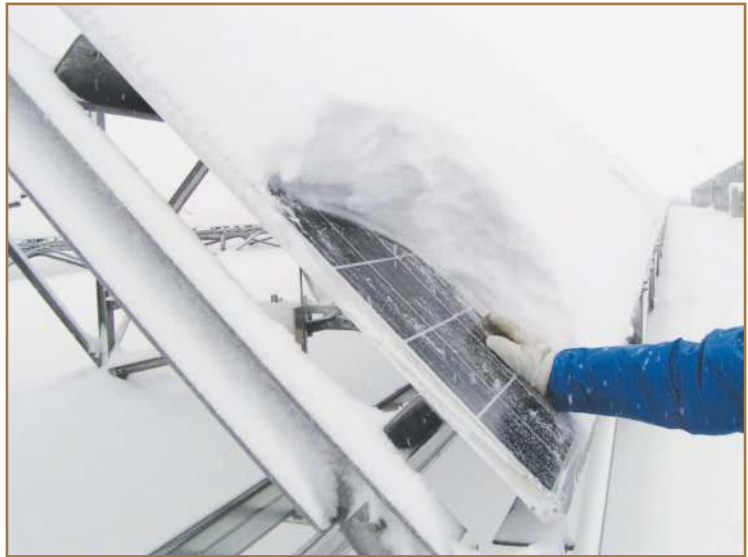
figure 14. Snow accumulation on the PV array.
