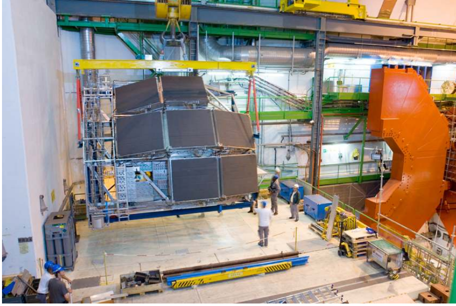
Figure 3.55: View of the seven modules of the HMPID mounted on the cradle.
