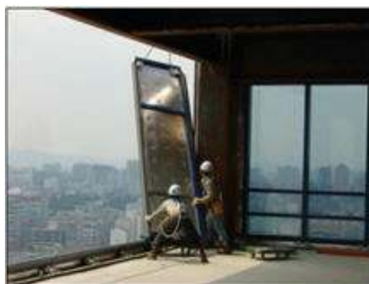
Fig. 2. Curtain-wall installation by human power
