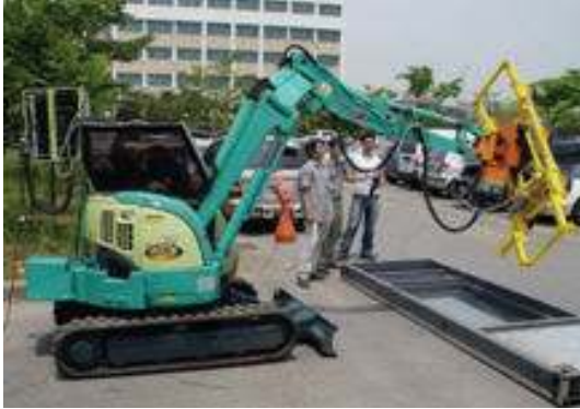
Fig. 3. Curtain-wall installation robot
